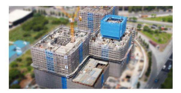
GTP100 Automatic hydraulic climbing formwork system is a construction technique that includes the climbing bracket, formwork, platform system, and suspension bracket, which are attached to the concrete structure. Once the formwork is stripped off from the shaped concrete, it driven by the hydraulic cylinders and guided by the climbing rail, the brackets climb up to the next level, repeating this cycle for the construction process.
